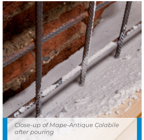
Pouring Mape-Antique Colabile into formwork
