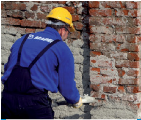
Application of PoroMap Rinzafo Plus with a rendering machine
