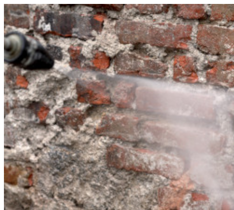
Powerwashing of the masonry
