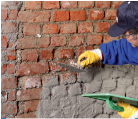
Application of PoroMap Rinzafo Plus with a trowel
