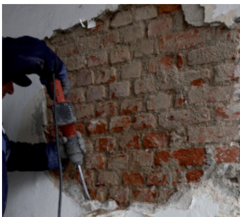
Removal of damaged render
