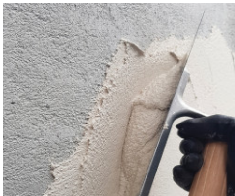
Application of PoroMap Finitura Granello on cured render
