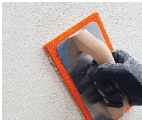
Finishing of PoroMap Finitura Granello with sponge float
