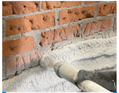
Application of Mape-Antique NHL ECO Risana with a rendering machine
