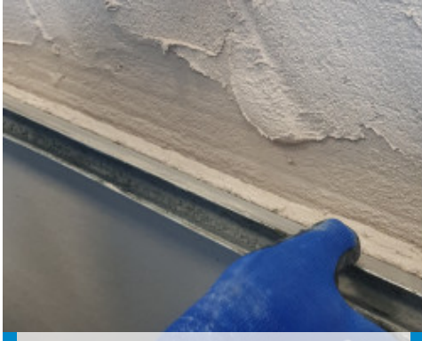
Flattening the surface of Mape-Antique NHL ECO Risana with a straight edge
