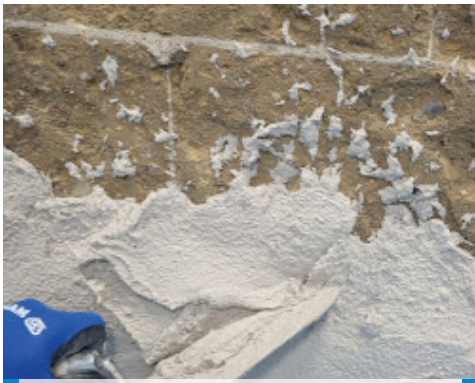
Application of Mape-Antique NHL ECO Risana with a trowel on tuff substrate
