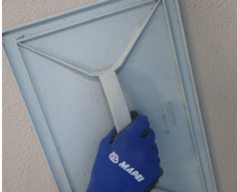
Levelling off Mape-Antique NHL ECO Risana
