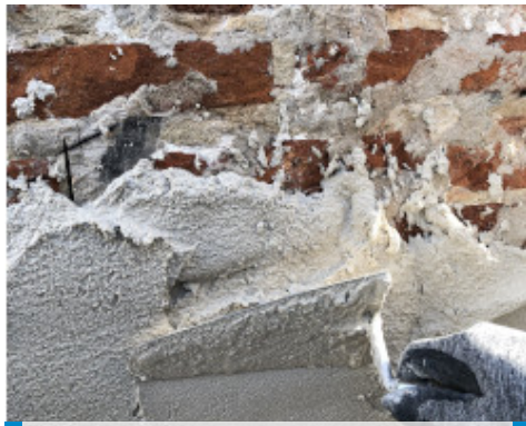
Application of Mape-Antique NHL ECO Risana with a trowel on brick substrate
