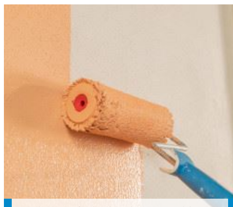
Painting of rebuilt substrates with Mape-Antique NHL Eco Restaura
