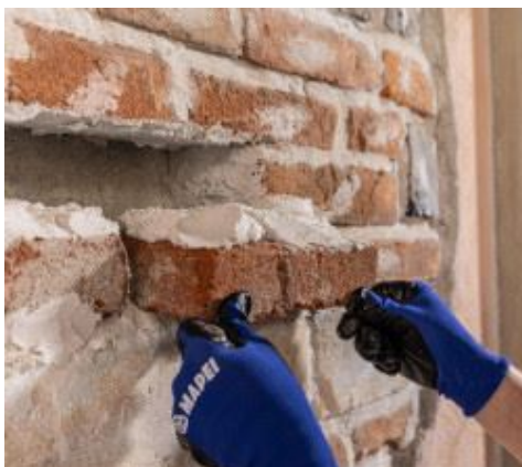
Rebuilding brick masonry
