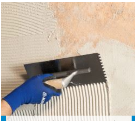
Application of the first skim coat of Antique NHL Eco Restaura
