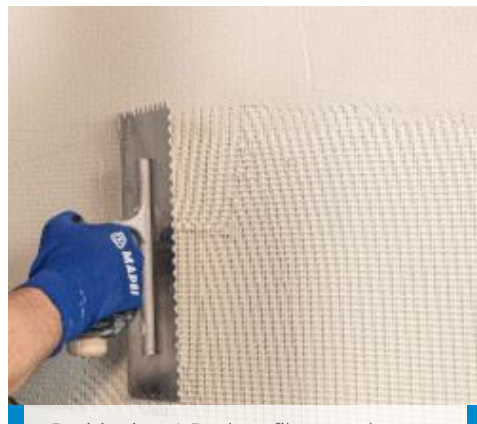
Positioning A.R. glass fibre mesh on the first skim coat
