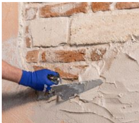
Levelling off and repairing render
