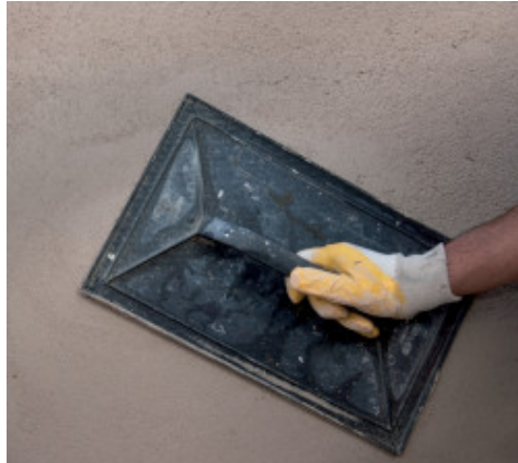
Levelling the render
