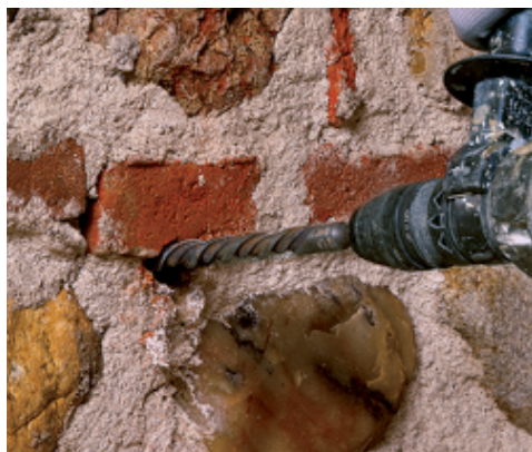
Making holes for Mapenet EM Connector
