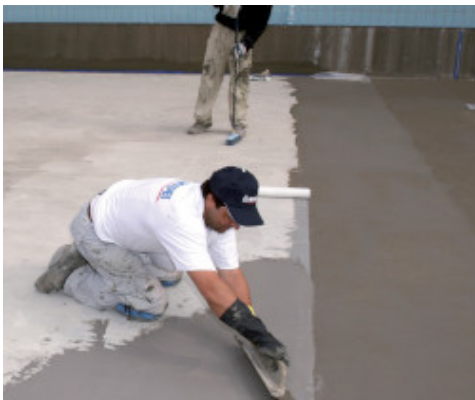
Waterproofing a swimming pool with Mapelastic Zero
