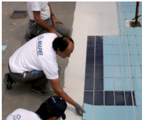
Application of ceramic coating on Mapelastic Zero
