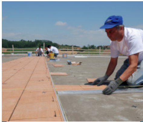
Laying ceramic tiles with Kerabond + Isolastic
