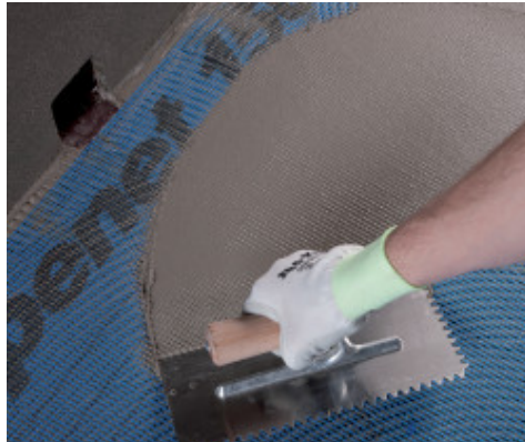
Application of Mapelastic Zero on Mapenet 150
