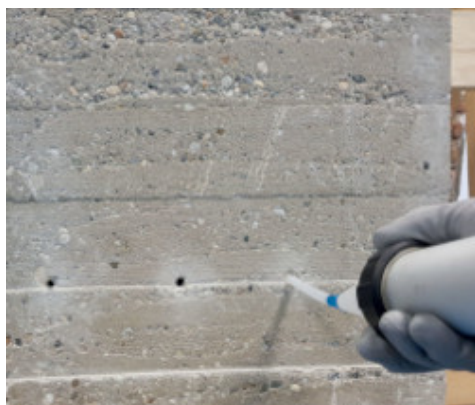
Create a chemical barrier in a concrete wall
