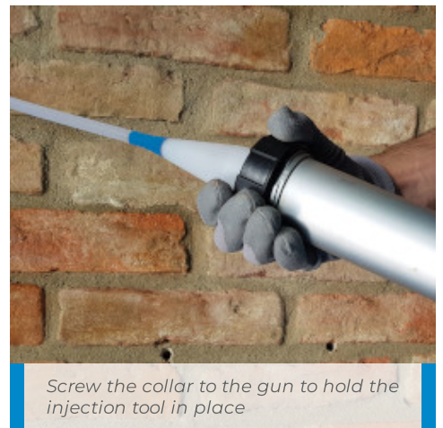
Insert a sausage in the extrusion gun and then cut the edge of the sausage on the side where the collar is going to be secured
