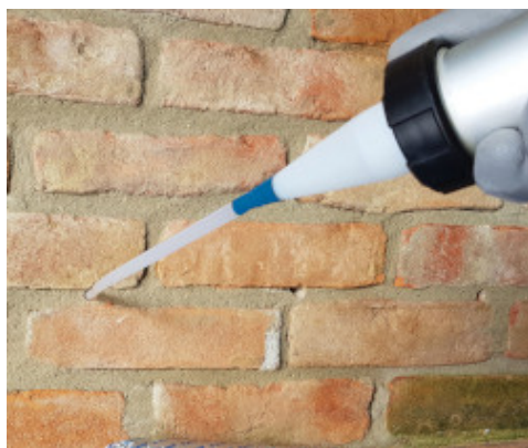
Extrude the cream in the sausage from the gun and fill all the holes
