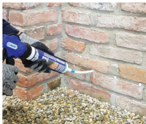
Extrude the cream from the cartridge filling each hole
