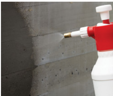
Application of Planiseal WR 100 by spray
