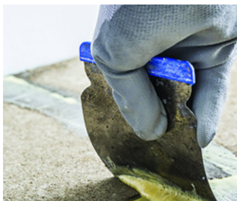
Spread the product evenly to fill the crack
